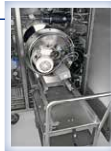
Detail technical area
